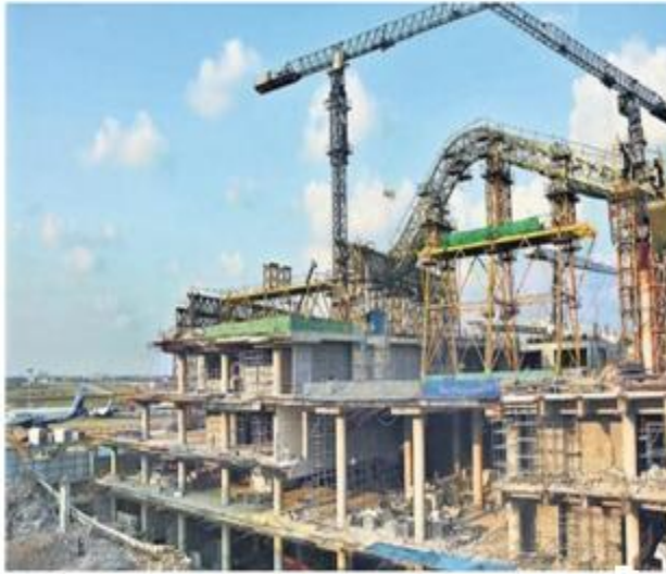
Construction activities in Chennai International Air port
