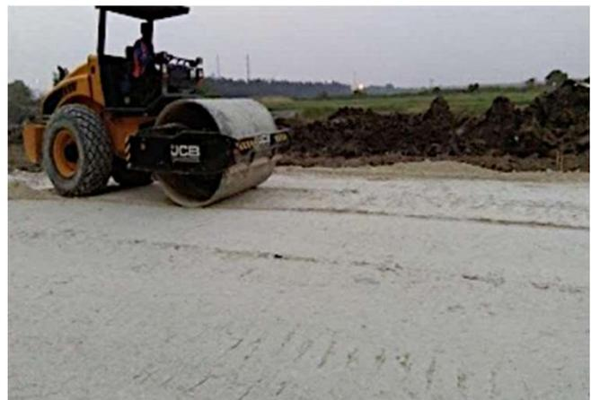
Compaction of Neutralised phospho-gypsum layers
