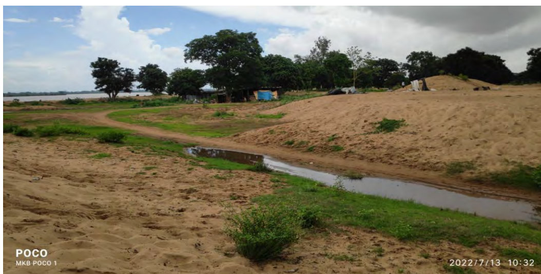
Figure 8: Low-lying silted storm drain between two elevated dumps of sand.
