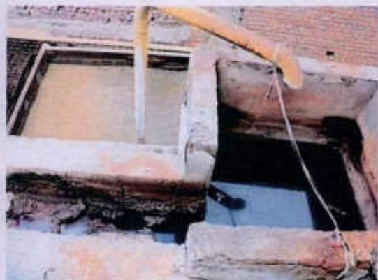
**Plate-8: Photograph showing the components of ETP lying defunct**
