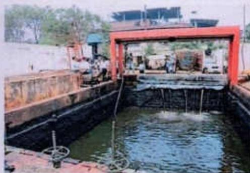
Plate-10: Photograph showing untreated effluent collection tank
