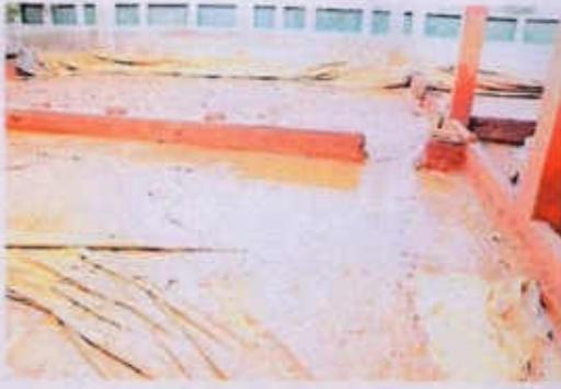
**Plate-11: Photographs showing the sludge being dried in the Sludge Drying Beds**
