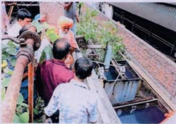
**Plate-7: Photograph showing the components of ETP lying defunct**
