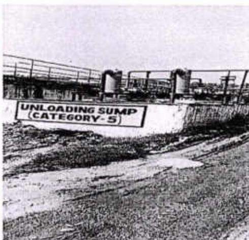
**Plate-1 : photograph showing collection and reaction tank for category 5 effluent (Electroplating effluent)**
